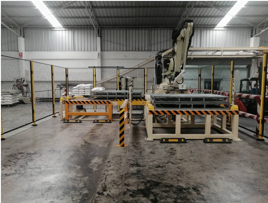
COMPANY : UNITED FLOUR MILL ( Line P8 )
